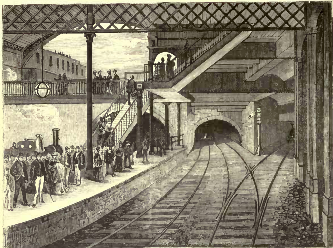
KING'S CROSS UNDERGROUND STATION IN 1865. (See page 227.)
